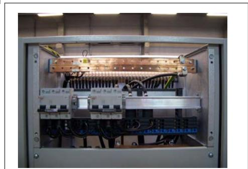
If an alarm is required for AC output breakers, a help contact attached to each individual breaker is used (OF or SD). The alarm function is common and uses one of the digital inputs on the control unit. The help contact limits the breakers quantity.
