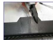
Cut holes to allow cable access
